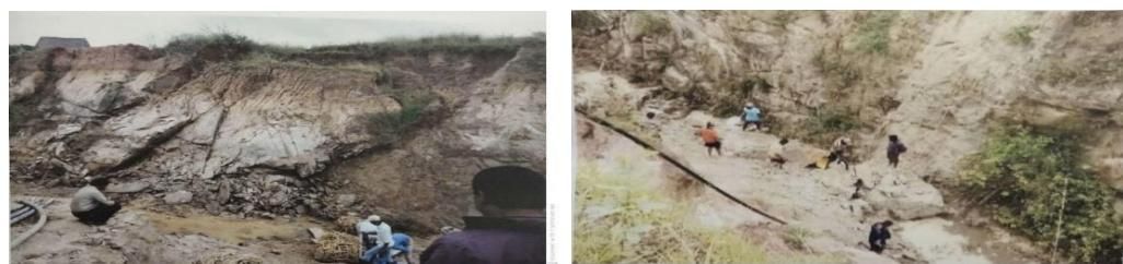
Fig No 8: Photos of non-uniform canal section
